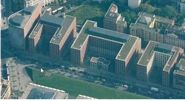
Fig. 4: Oblique view aerial image of the building under investigation (© Microsoft® BING™).
